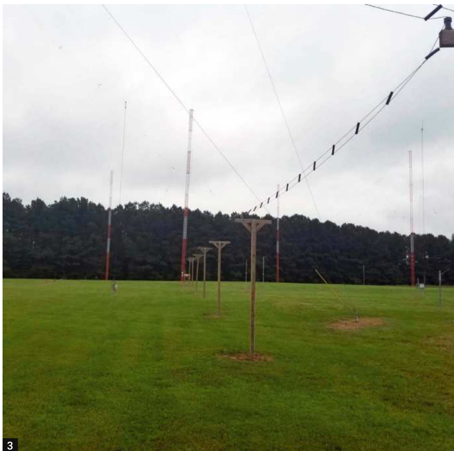
Fig. 1: The remote receiver system: All SDR, with analogue backup. Fig. 2: The entrance to the 'ON AIR' studio. Fig. 3: This is the open wire feed line to a 600-metre skywave loop antenna.
